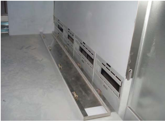
Ventilation slots at the bottom level of an elevator car
