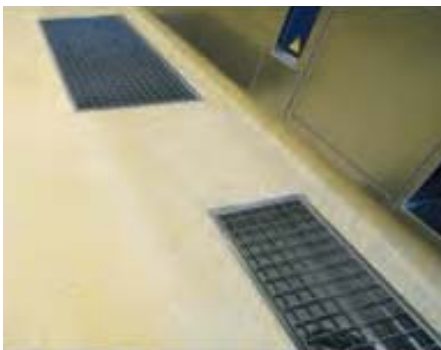
Floor drains in an elevator lobby
