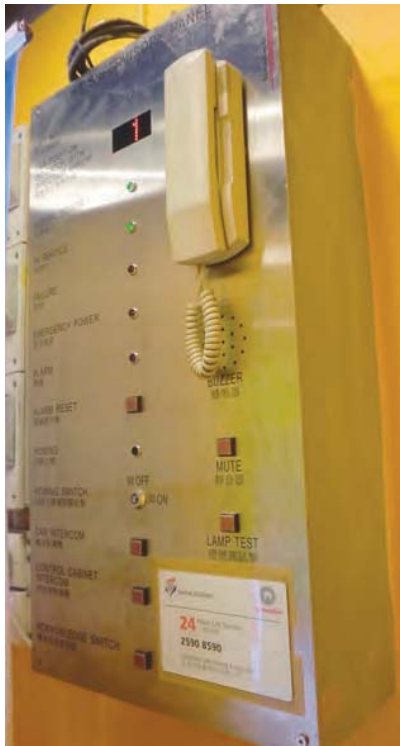
All centralized monitoring and communication systems require a protected power supply. These images show elevator supervisory systems that require an emergency power supply.
