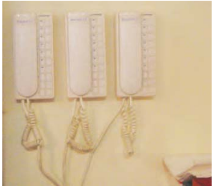
Centralized intercoms must be labeled for clear identification of the calling elevator.
