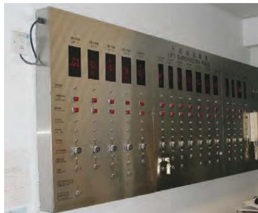
A large supervisory panel with a centralized intercom system
