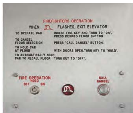
Typical arrangement of a Phase 2 Firefighters' Emergency Operation unit
