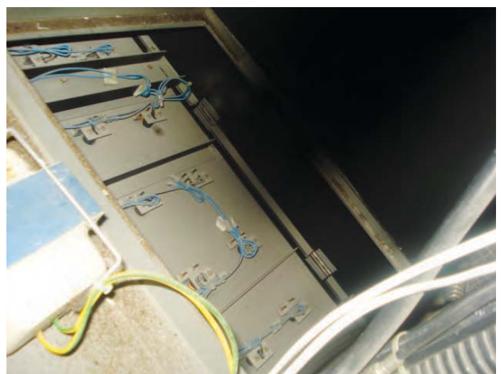
Escape hatch on an elevator car roof permanently blocked by the car's suspended ceiling
