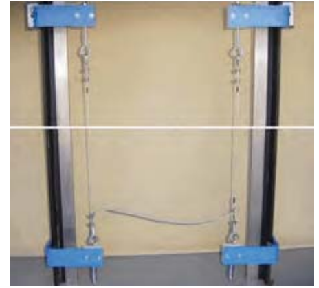
A typical counterweight derailment switch
