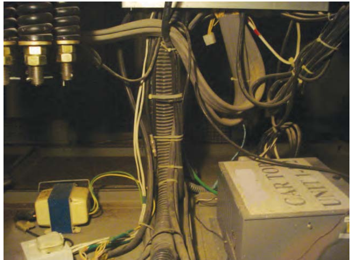
Local modification to factory-supplied lighting is not recommended.
